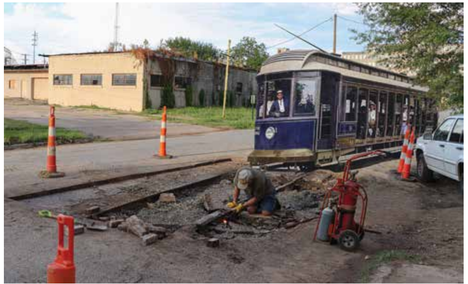
(above) Streetcar conductor looks on as Frank Head works feverishly to cut the streetcar track before it is covered back up forever.
